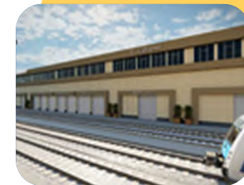
6 -Strengthening and repair
